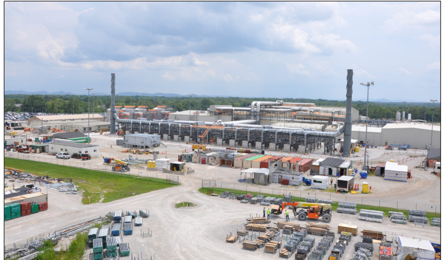
Blue Grass Chemical Agent-Destruction Pilot Plant in Richmond, Kentucky.
